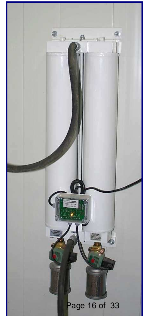
Twin Tower Drier dries air to minus 10 dgr
