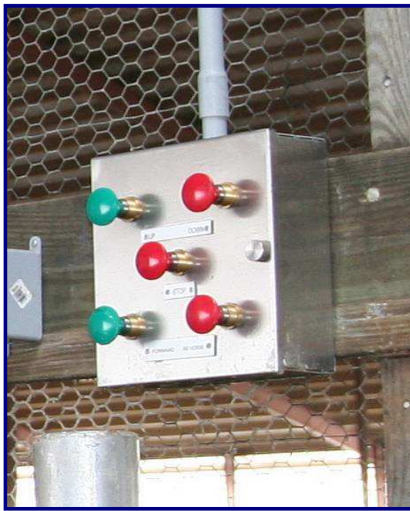
Center: Remote Controls in back of Holding Pen
