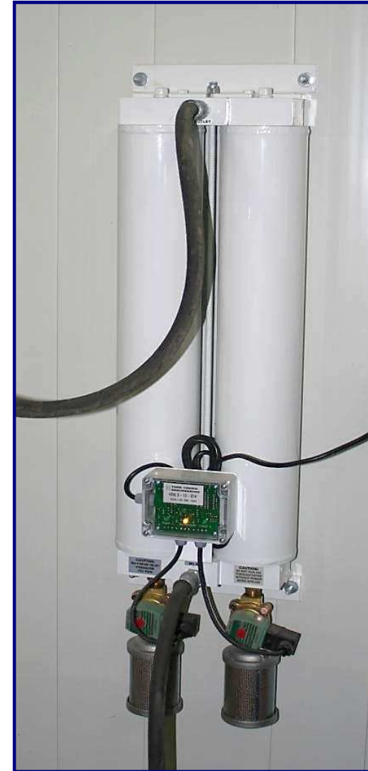
Twin Tower Drier dries air to minus 10 dgr
