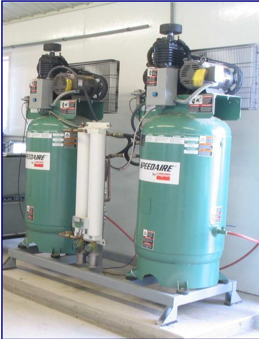
(2) 5 hp Speedair Compressors, modular, Page 17 of 33
