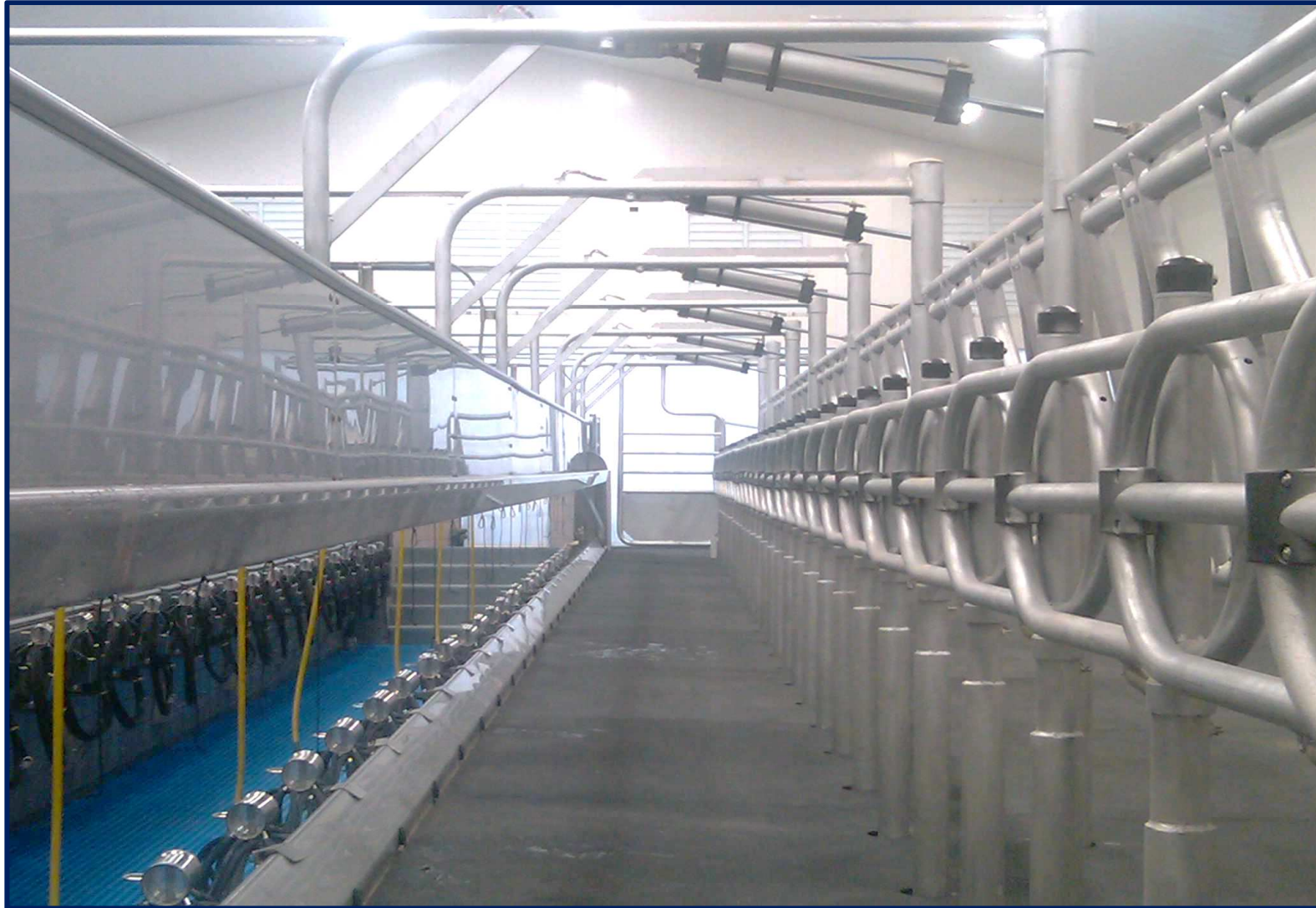
DeLaval Dbl. 30 Parallel installed near Green Bay
