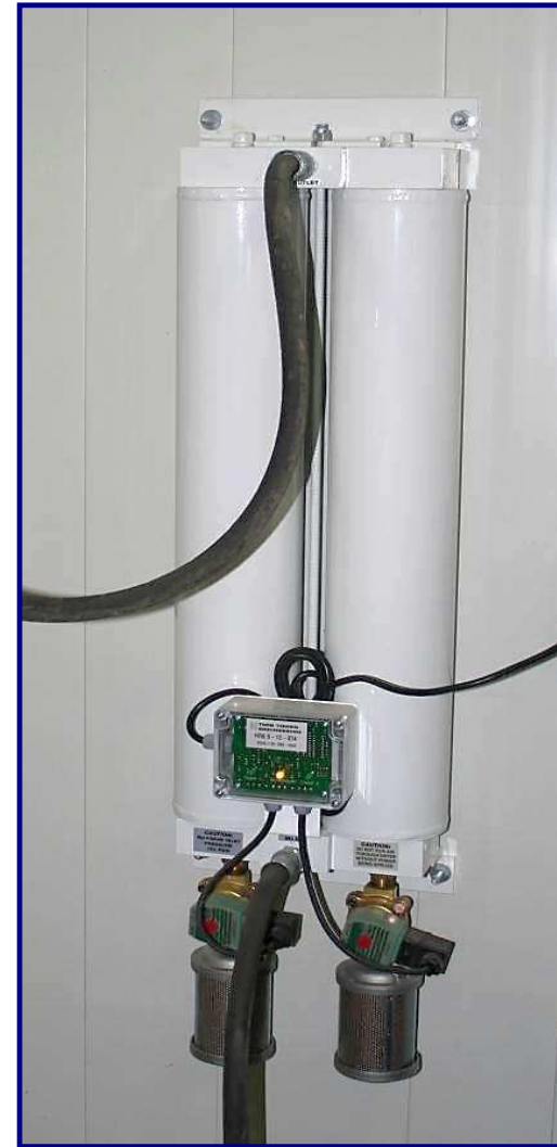
Twin Tower Drier dries air to minus 10 dgr
