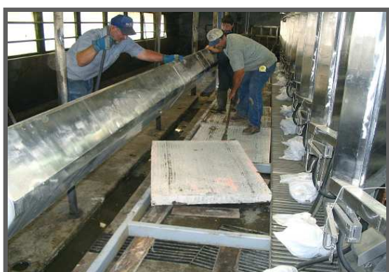
Each slab was cut a week ahead of time, numbered and cross referenced to its designated place.
