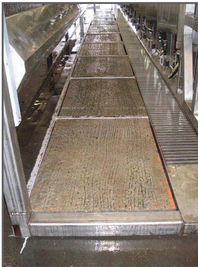
Ready-to-go cow platform one hour after parlor had been placed. Slabs will be replaced later on with poured concrete
